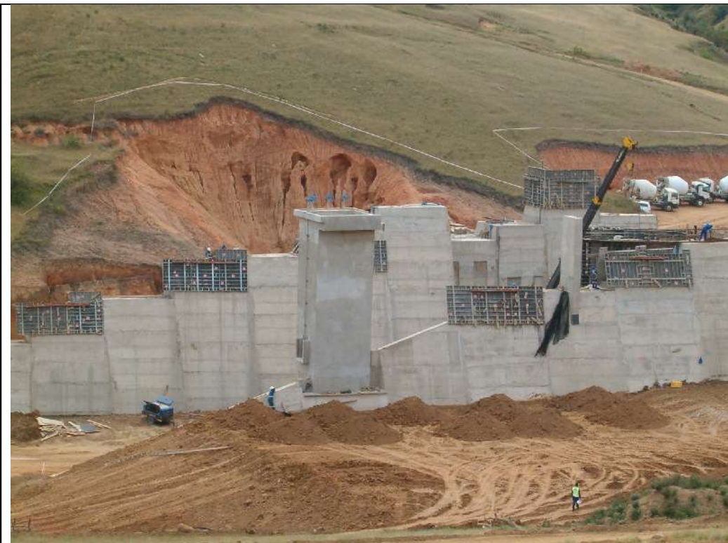
Mhlabatsane Dam near Highflats, KZN. (Umgeni Water)
